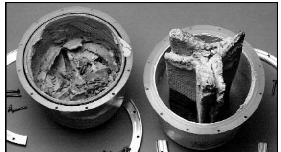
Figure 23-1. Tank filled with mineral buildup.
